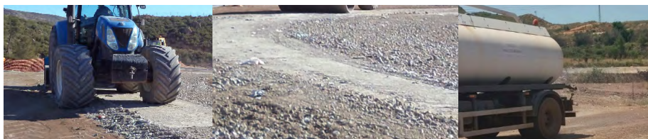
Image 1, 2 and 3. Extended, compacted and crushed debris irrigation.
