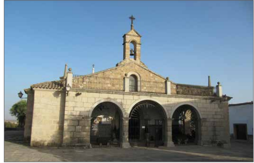
Portada, fachada principal
