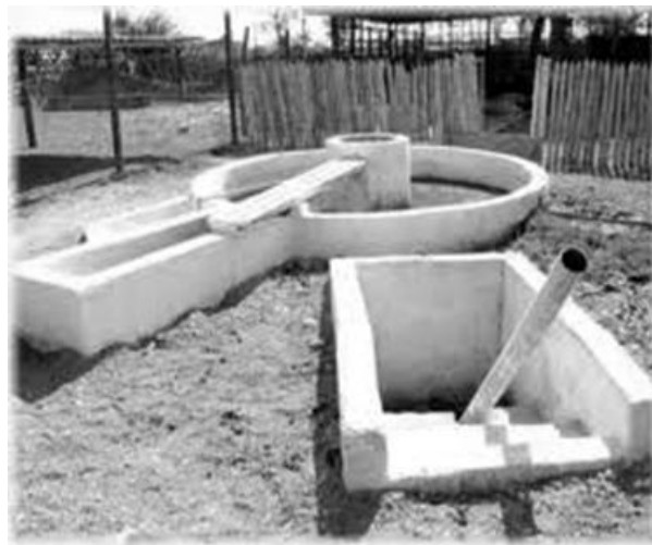
Image 2. Plant Fixed Dome. Web image. F. Cut Problems of Biogas Technology. Cuba, CUBASOLAR (No. 36, December 2006). Available in: http://www.cubasolar.cu/biblioteca/energia/Energia36/HTML/articulo04.htm
