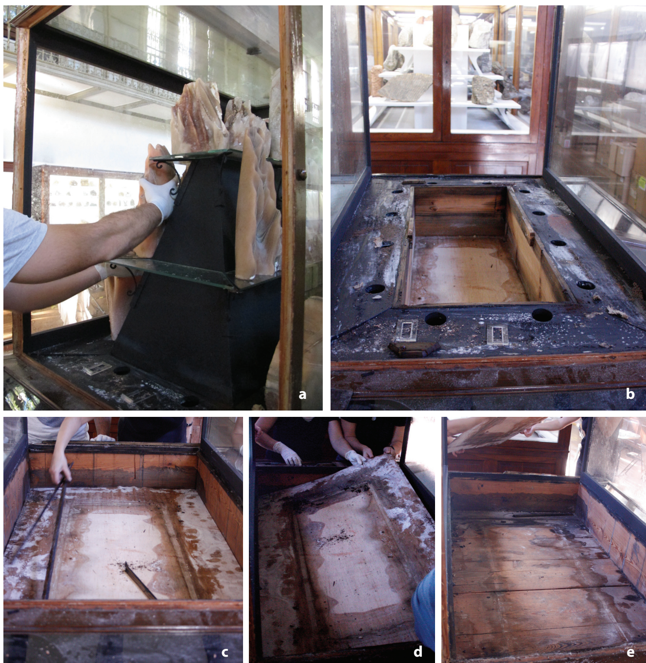
Figure 5.- The dismantling of the showcase. a: removal of the specimens after their original positions were recorded. b: after the removal of the display pyramid, the highly degraded inside of the showcase, greatly affected by the humidity, became apparent. c: a sheet protecting the wooden struts supporting the base was removed. d and e: the base of the showcase had also greatly deteriorated (D. Fernández – MCNB).
