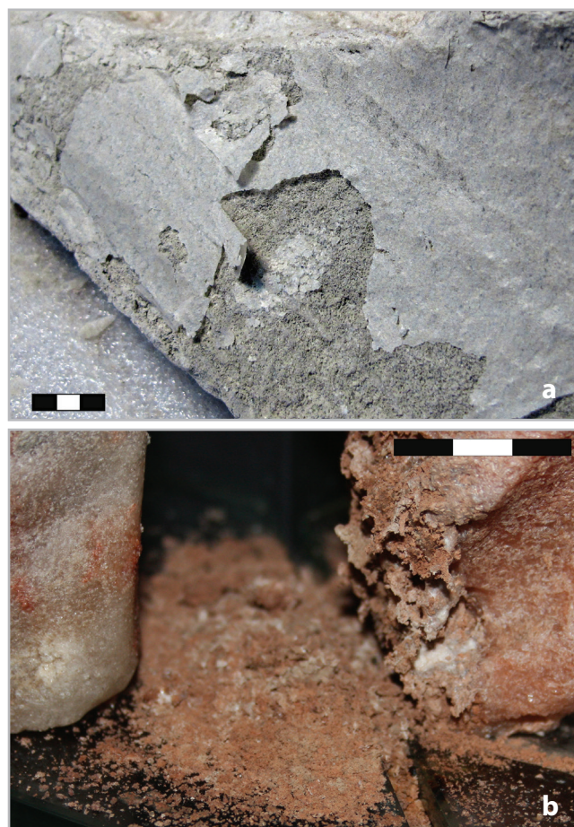
Figure 3. - Detail of the condition of the saline specimens before work began. a: example of flaking. b: one of the rocks affected by sanding (M. Pérez – MCNB).
