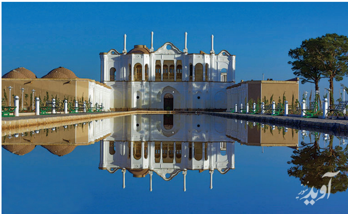
Figure 15: Fathabad Garden, Kerman, front view of the main building. (Photo by: Hamid Sadeghi, 2015)
