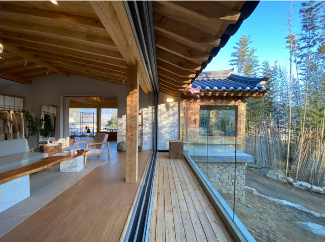
Traditional and modern rafters | Cabios tradicionales y modernos | Caibros modernos e tradicionais (Youngchae Park)
