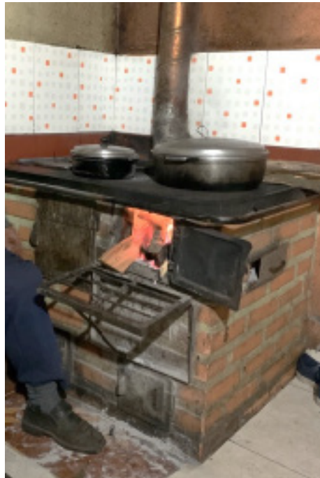
Figure 2. Stove in Operation with the Firewood Flap Open
