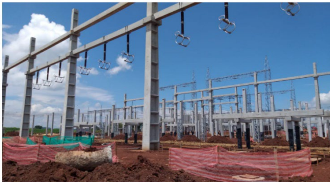
Figure 2. Itá-SC substation during expansion. Source: Authors' own production
