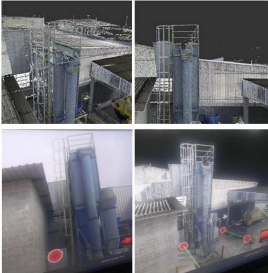
Figure 3. Point cloud environment obtained through laser scanning.
