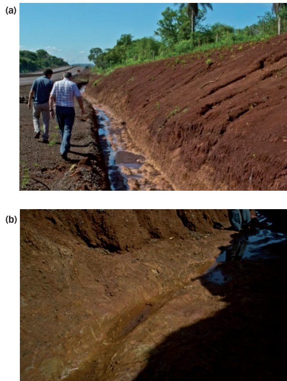
Figure 11: Progressive Field 6,200; (a) Profile of the counter slope in the cementation process and (b) Slab in the natural cementation process.
