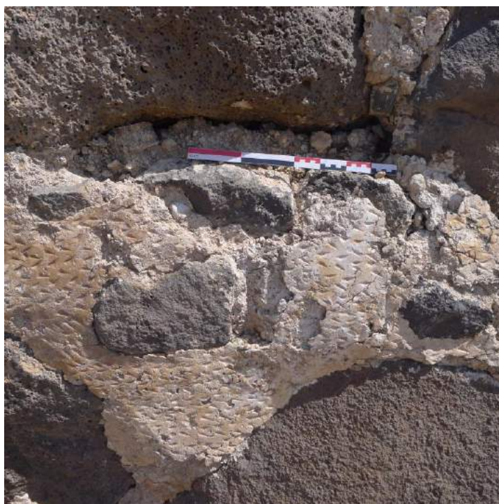
Fig. 3 – Construction of cyclopean blocks, with joints of plaster with scale-shaped incisions. (© L. D'Agostino).
