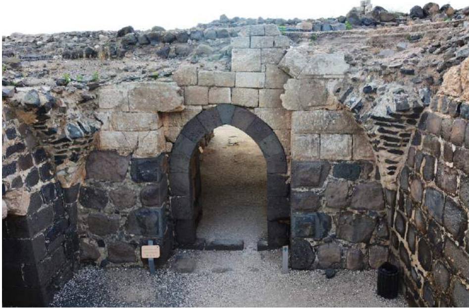
Fig. 2 - West door of the inner building; basalt embankment and upper siding in limestone. (© L. D'Agostino).
