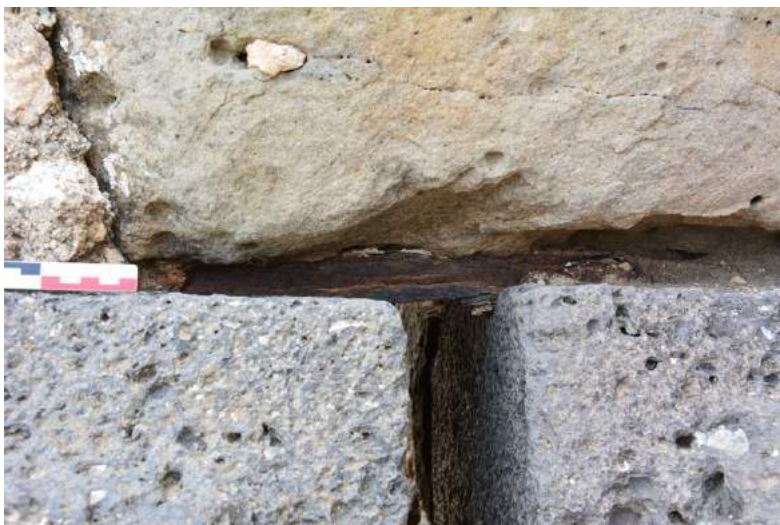
Fig. 10 – Staple disposed under the lintel of an arrow slit. © L. D'Agostino.
