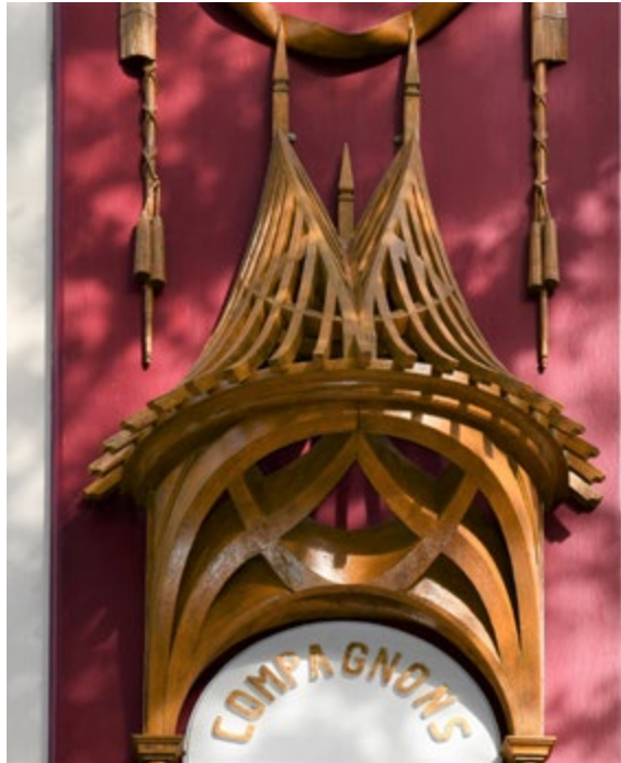
The façade of the Aux Arts et Sciences réunis restaurant at 161 avenue Jean Jaurès in Paris features a small guitarde canopy with a double-curved surface that has been sectioned on an angle to create two double-curved hips and a straight valley in the center (Sim Ayers)
