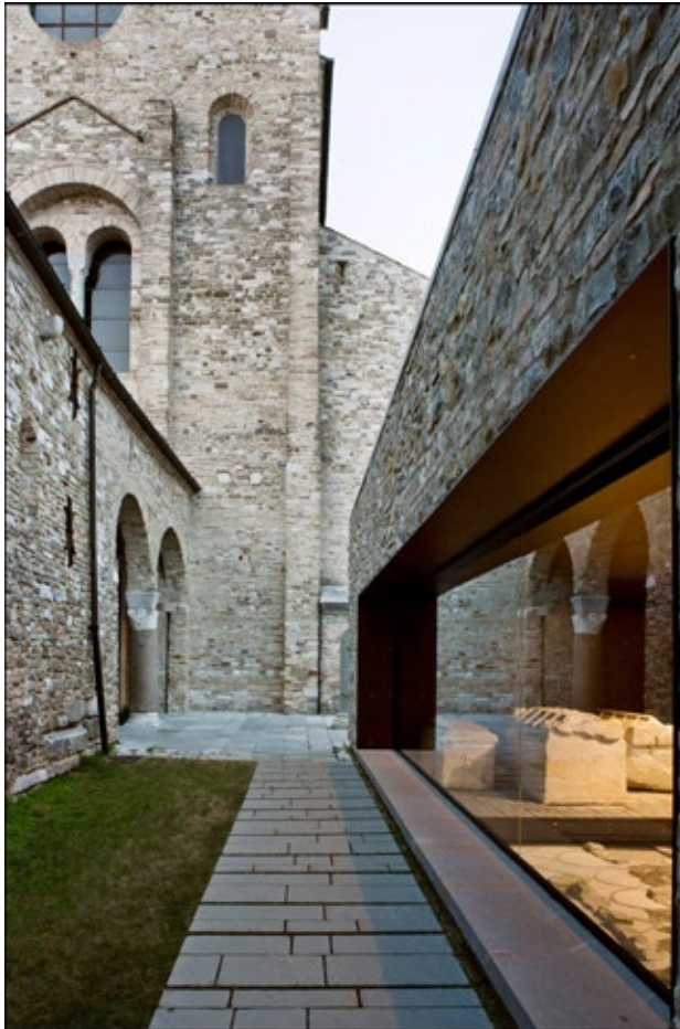
[Fig. 13] Aquileia (Udine), the new south hall of the Baptistry of the Aquileia Basilica. Manuela Castagnara Codeluppi, Giovanni Tortelli e Roberto Frassoni . Architettura, storia e memoria (Milan: Electa, 2019).
