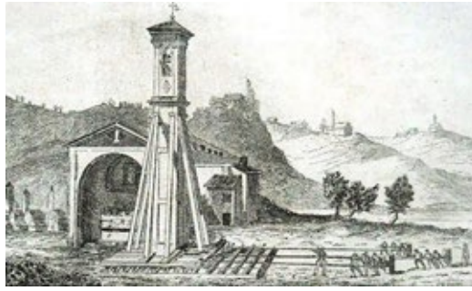
[Fig. 3] Crescentino, moving the bell tower in a nineteenth century etching. Maggiobello, Ex situ , 2010-2012.
