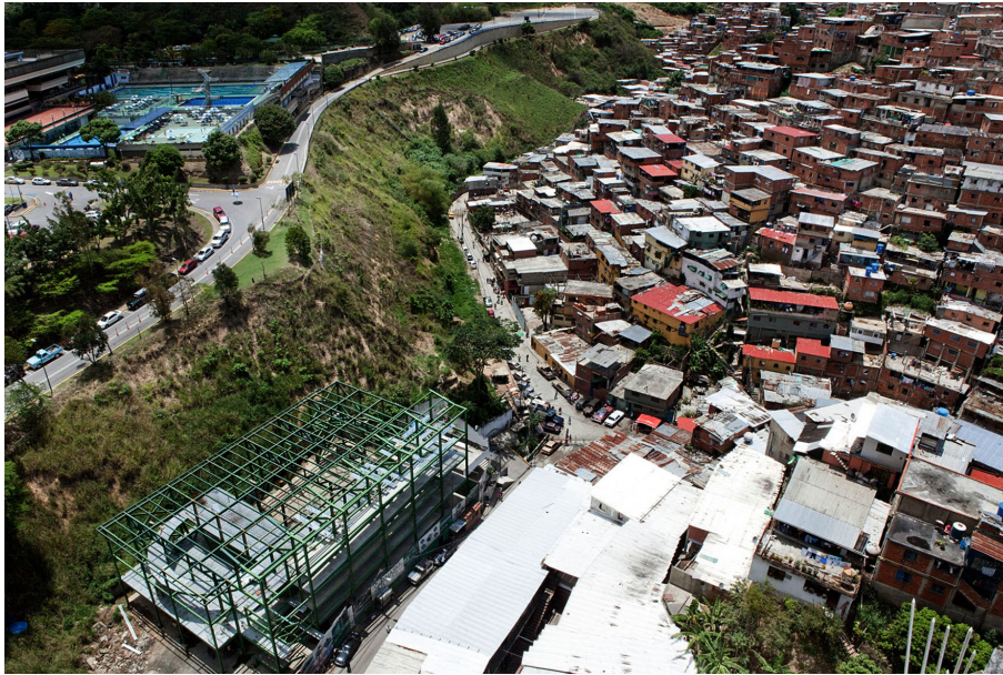
Image 3 - UT-T. Vertical Gym.Construction
