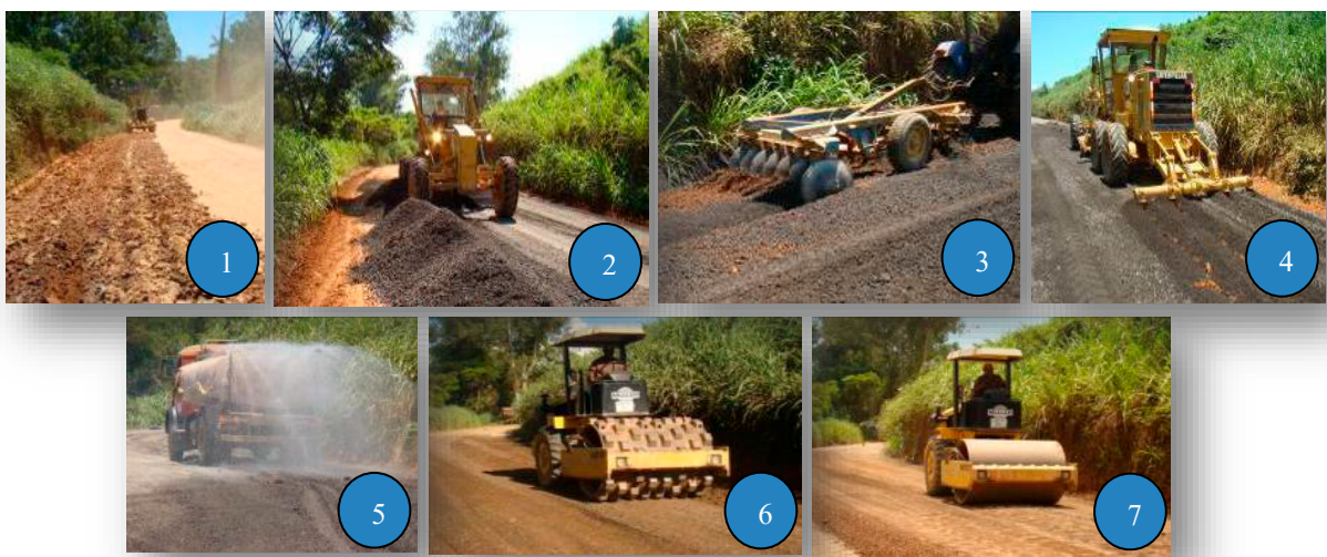
Figure 1. Application of the aggregate compound on a rural road
