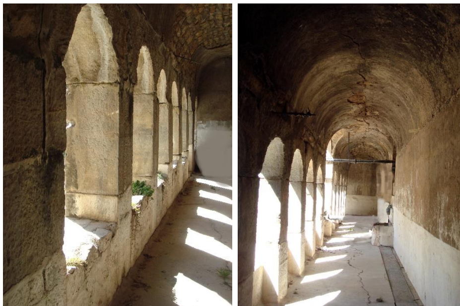
Figure 5. View of the courtyard on the North & South side, today a passage to reach the fountains, another time a paved pipe where circulated the drawing water. © MAHDADI, N. 2020.
