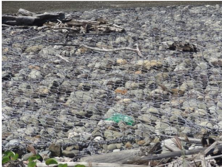
Figure 2. Airport Sector: Installation of gabions. Taken in the field on December 6, 2017.
