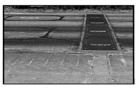
Figure 3. WIM system of flexible bands [35]
