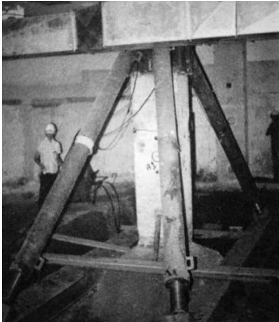
Figure 7. Foundation reinforcement at Paulista Mall ([2])
