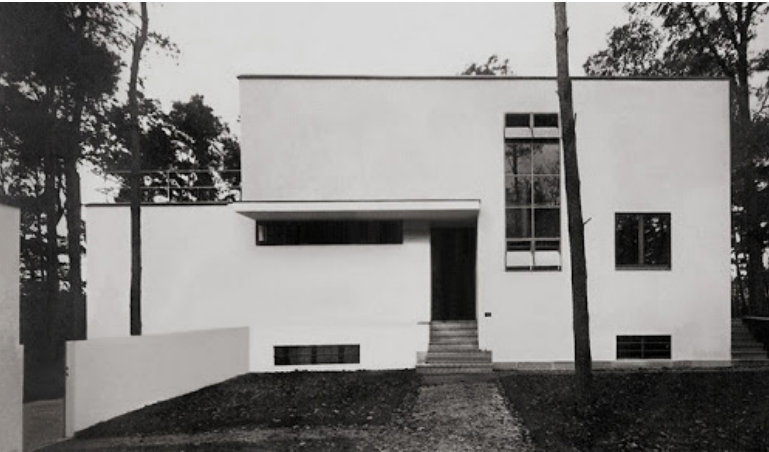
Figure 7. Director's house, Bauhaus, Dessau, Germany, Walter Gropius, 1925-1926: A formal type that became the founding imagery for a new tradition (Postcard)
