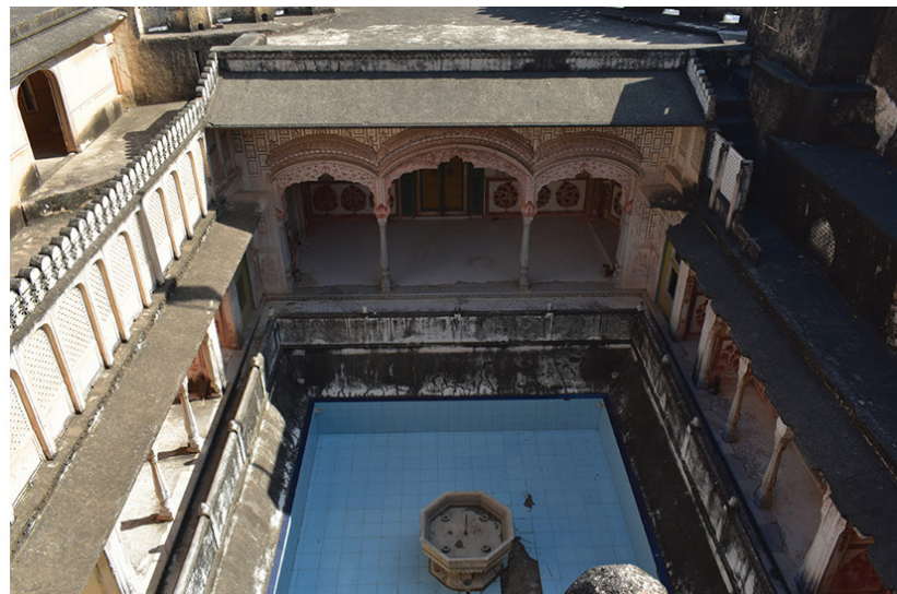
Figure 6: Traditional lime plaster replaced by ceramic tiles in the pool of Sunheri Burj, in the Ranvas at Kuchaman Fort: (A) Original materials used in construction (kuchamanfort.com); (B) Poor conservation practices
