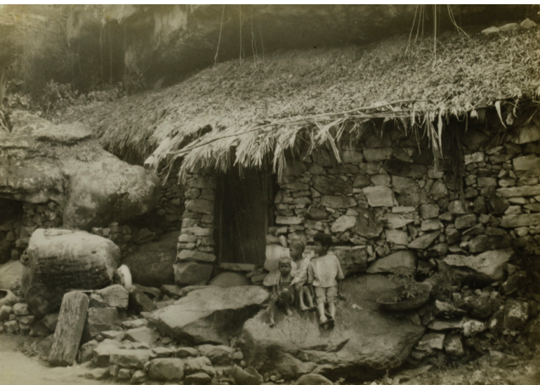
Figure 5. Miners' house Built under the stone vault with dry stone technique, Mucugê, state of Bahia, no date (IPHAN Digital Collection)
