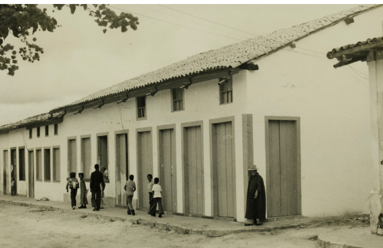
Figure 6. Residential ensemble of Direita do Comércio street, Mucugê, state of Bahia, 1978 (IPHAN Digital Collection)
