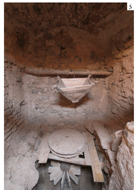
1: The main chamber after its excavation 2: The storage chamber after the roof construction 3: The main chamber after its excavation 4: The wheel reassembling at the main chamber 5: The wheel once it was reassembled (Sonia Beygi)
