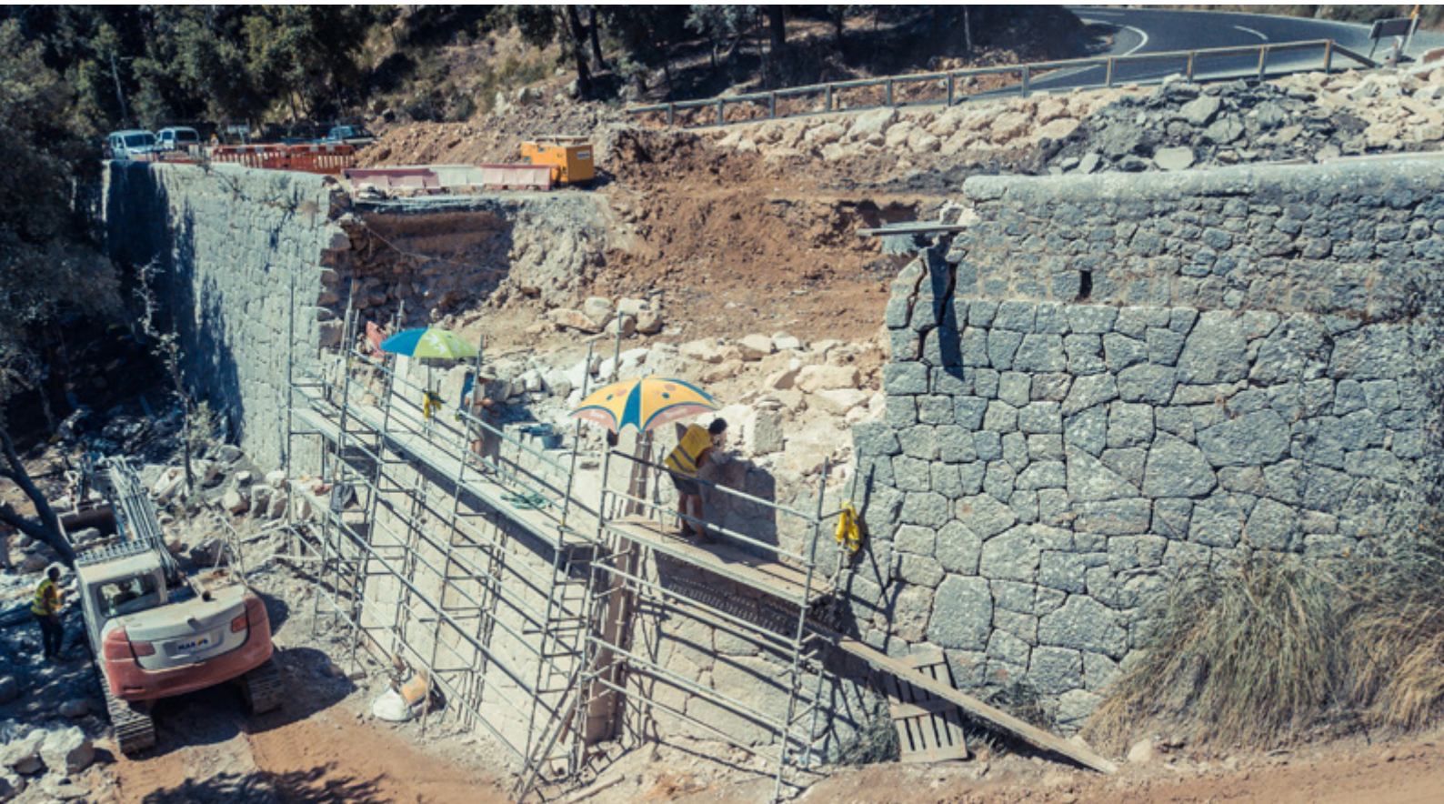
Reconstruction of the dry stone wall | Reconstrucción del muro de piedra seca | Reconstrução do muro de pedra solta (Born To Sea Media)
