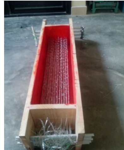
Figure 1. Wooden molds within aluminum accessories and PET-profiles matrix: 5 layers with 11 threads every layer. Source: The authors.
