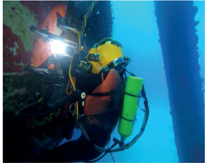
Figure 1. Welder performing the underwater wet welding process [4].
