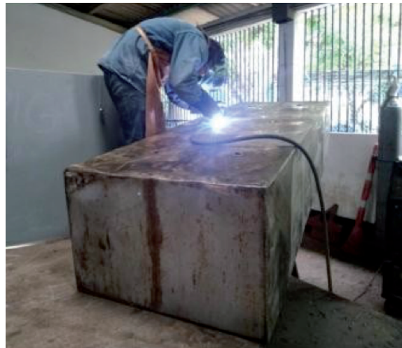
Fig. 3. Cutting and welding to fix check valve couplings.
