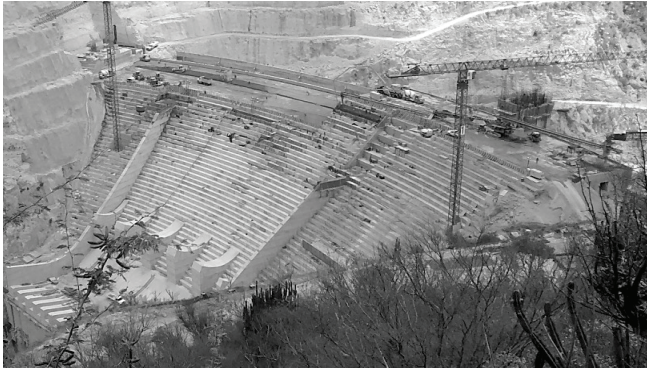
Figure 3. 79 meters of built height in the El Zapotillo dam. Source: The Authors.
