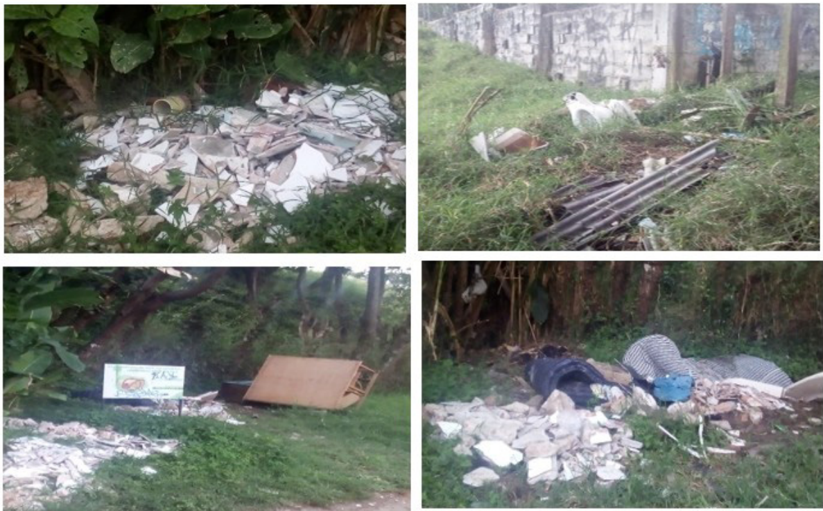
Figure 1. Inadequate disposal of construction and demolition wastes (C&D) in Colombia Source: own
