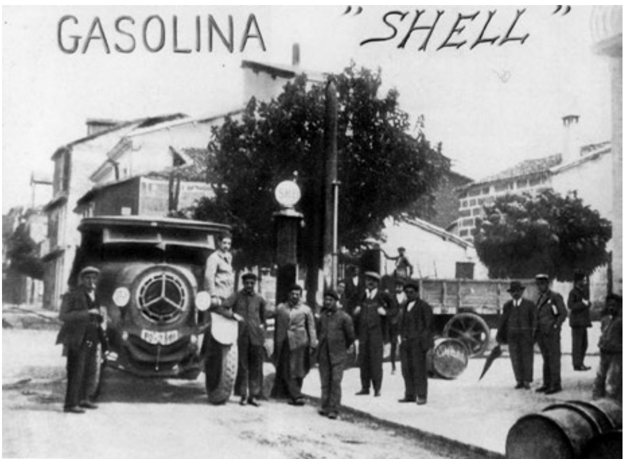
(1920 ca)-Gasolinera Cortés na Crt. Ribadavia
