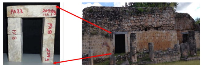
Figure 10. Schematics of archeological lintel as a horizontal structural part that is placed above across the opening. Source: Adapted from authors own information
