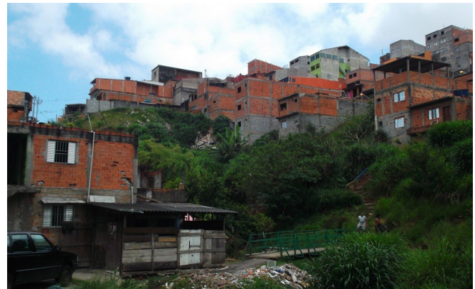
Figure 1. View of the school neighborhood from the school gate. The river runs under the bridge just beside the school
