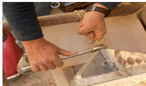
Figure 20. Application of the CFRP pre-tensioned wires.
