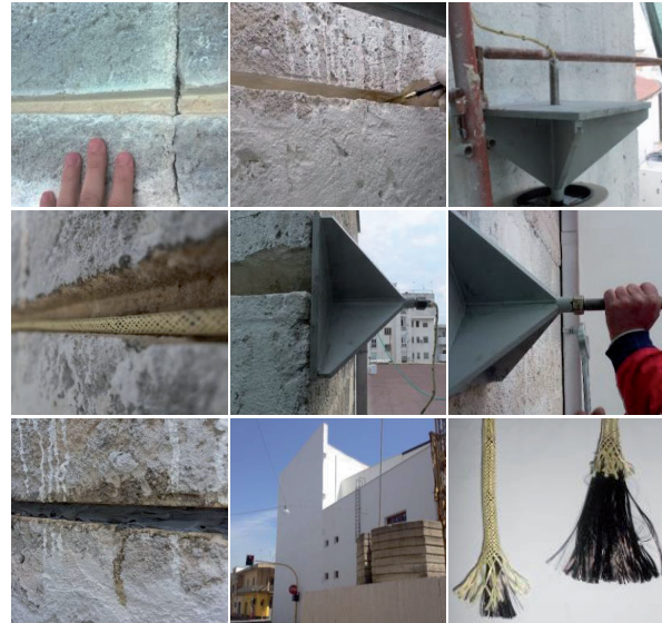
Figure 10. Process steps (1-11) and detail of the CFRP wire.
