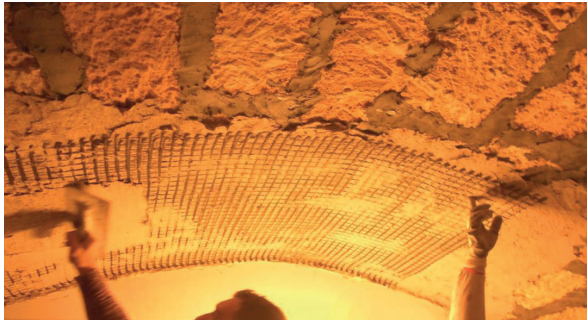
Figure 18. Installation of FRCM glass fiber system.
