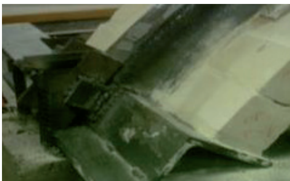
Figure 8. Shear restraint at the fixed abutment.
