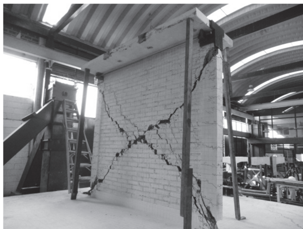
Figure 11. Cracking on the masonry wall the day after. Source: The Authors
