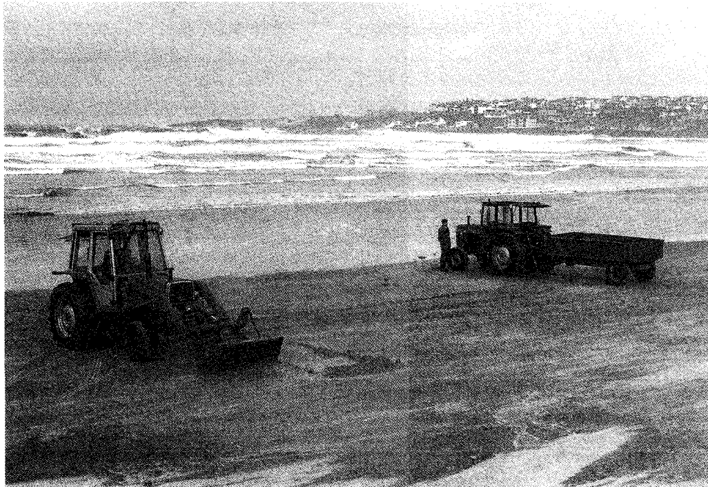
Figure 7a.- Sand Removal. Portstewart Beach
