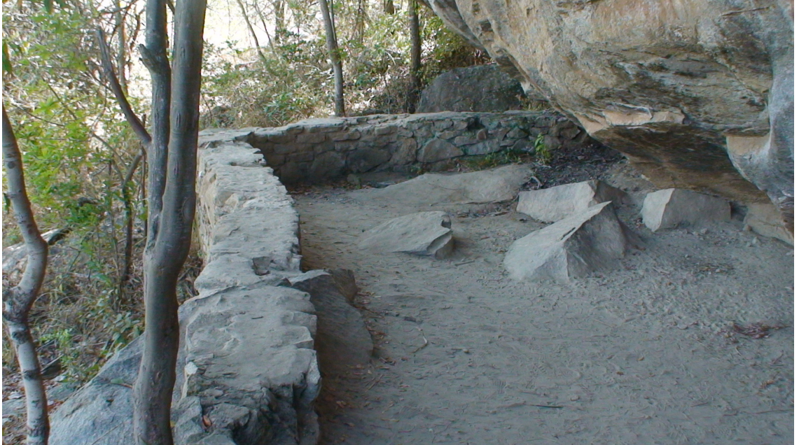
Plate 1: A wall stump that once was the base of a framed protection wire mesh at Site B1, Kolo (Photo by the Author, July 2012)
