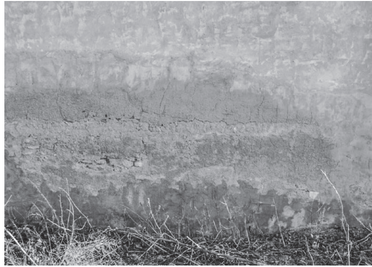
Figura 6. Revestiments inadequats
