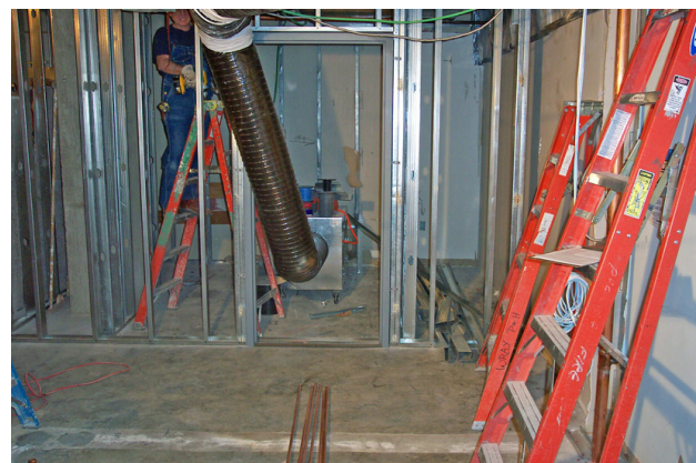
Fig. 8. Construction area showing HEPA filtration unit for dust control.
