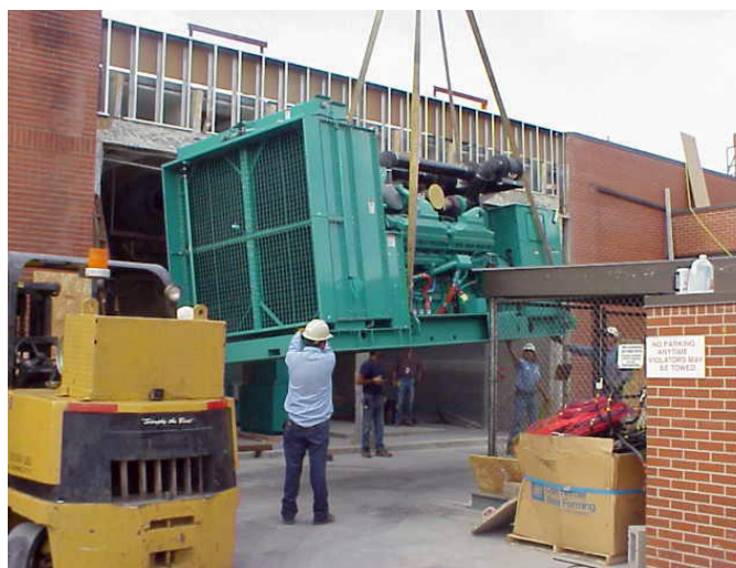
Fig. 2. Installation of one of a pair of 2500 kVA emergency generators.
