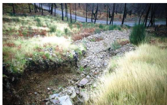
Photo 5 - Detail of the material deposited in the slope after gullying.
