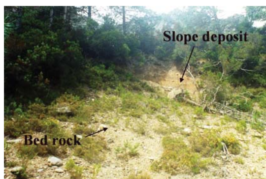
Photo 8 - Detail of the place where the debris flow of Portal da Freita began, whose failure is clearly related with the contact of the deposit with the bedrock.
