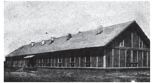
[Fig. 21] Panelized barrack (type Ш-11) – a dormitory for the single. Source: [Electronic resource] – Access mode: http://s16.photobucket.com/user/chmelnizki/media/Архитектура/Stalingrad_Doma_ASSR_N10-45-600_zps8a9525fe.jpg.html .
