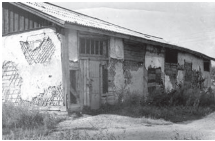
[Fig. 19] Township of first builders from Sergo Ordzhonikidze machine-tool plant of the Order of the Red Banner of Labour. Plastered up lathing plank barracks. Source: Поселок первостроителей ЗСО [Electronic resource] – access mode: http://eh-la-bas.livejournal.com/2398.html .
