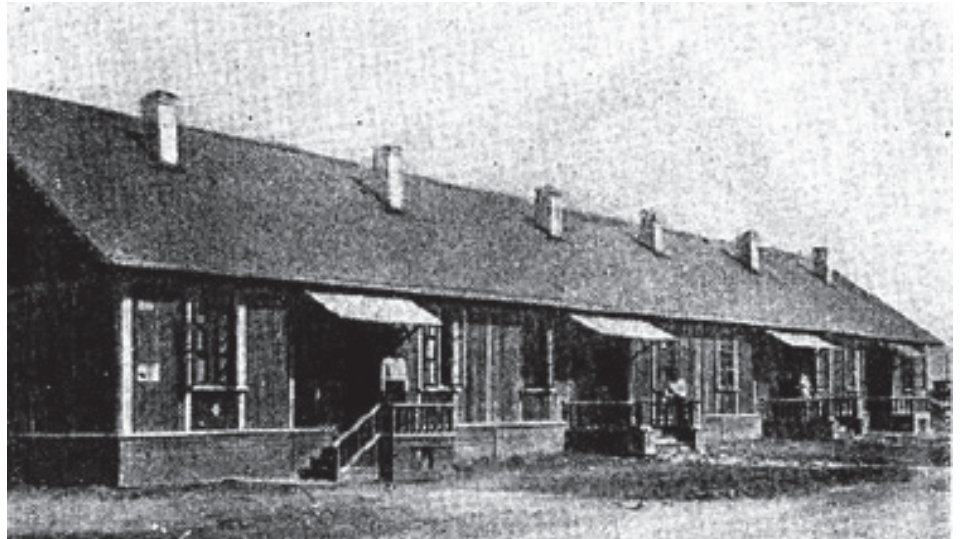
[Fig. 30] Panelized barrack (LJ-10 type) with separate rooms for families. Source: [Electronic resource] – Access mode: http://s16.photobucket.com/user/chmelnizki/media/Arhitektura/Stalingrad_Doma_ASSR_N10-45-600_zps8a9525fe.jpg.html .
