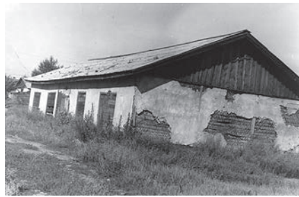
[Fig. 20] Township of first builders from Sergo Ordzhonikidze machine-tool plant of the Order of the Red Banner of Labour. Plastered up lathing plank barracks. Source: Поселок первостроителей ЗСО [electronic resource] – access mode: http://eh-la-bas.livejournal.com/2398.html .
