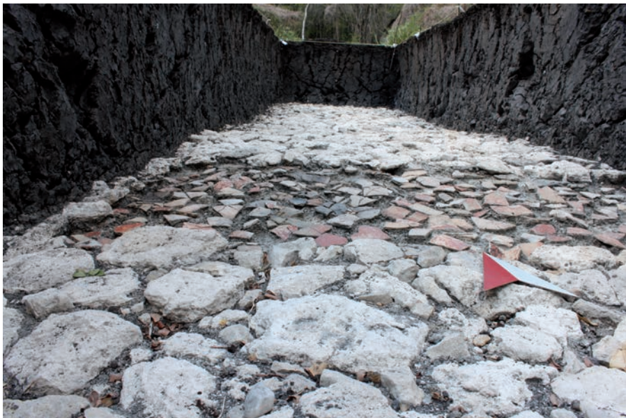
FIGURE 19. Pavement of limestone slabs at the bottom of the Aguada Oriental
