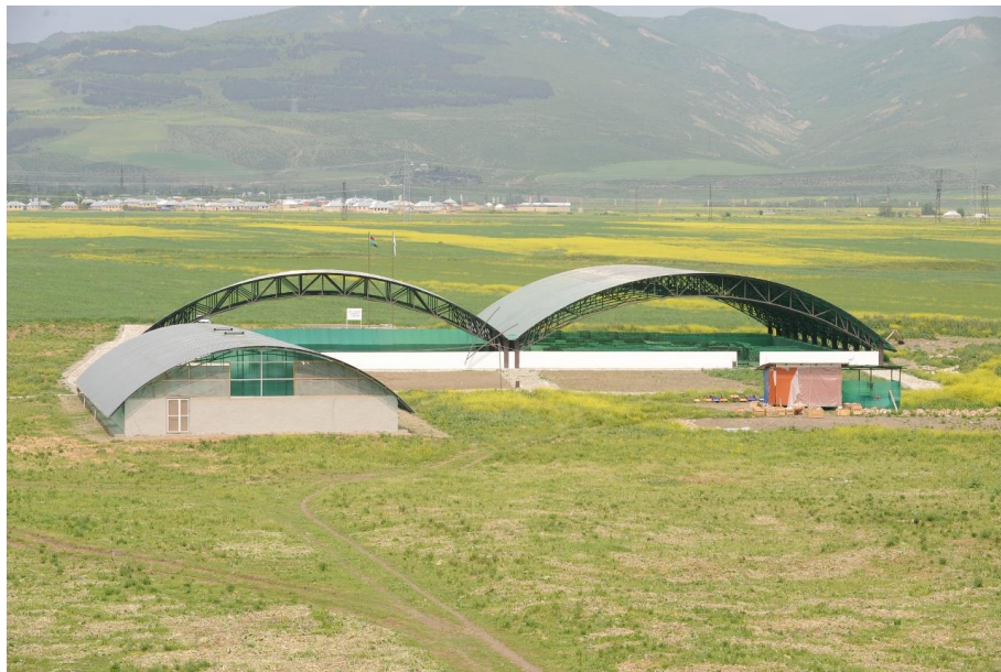
Fig. 8. Covering sites—3 rd and 4 th excavation site.
