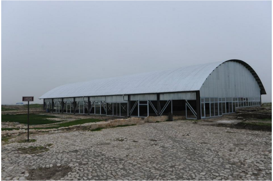
Fig. 7. Juma Mosque after covering.
