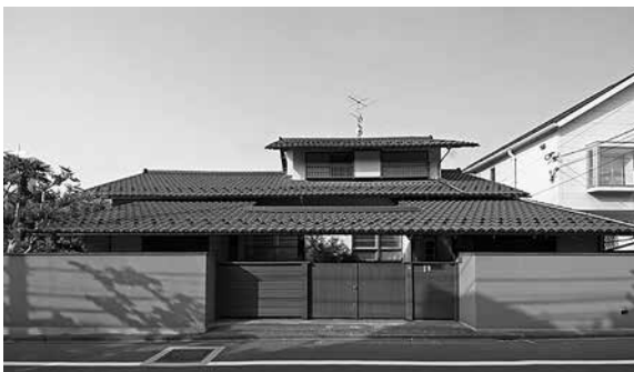
Fig. 19. Kasama House, Tokyo. Designed by Kunio Maekawa, 1938. Tokyo Architecture pictures: www.flickr.com/groups/tokyoarchitecture
