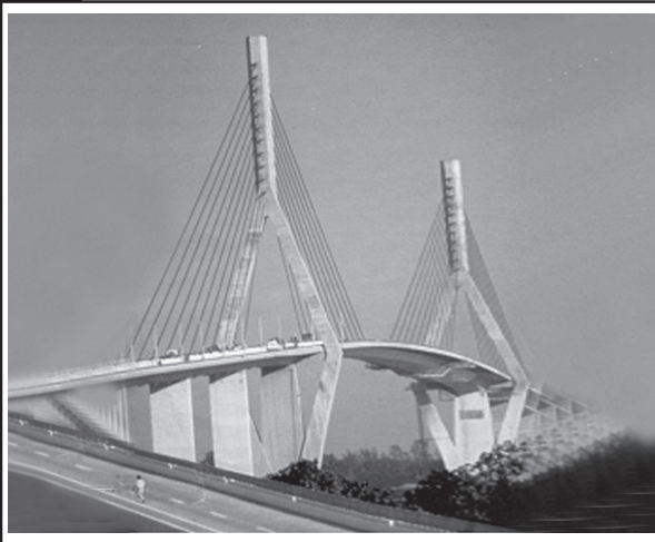
Figure 1. General view of Tampico bridge.
