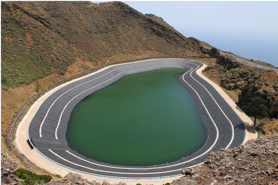
Figure 6: Water reservoir (Santamarta-Cerezal, 2013)
