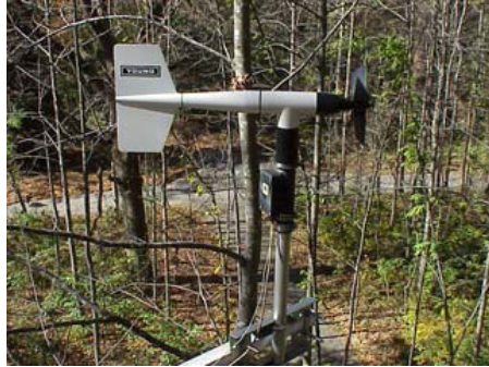
Figure 6. Anemometer and Wind Vane at 10 meters
