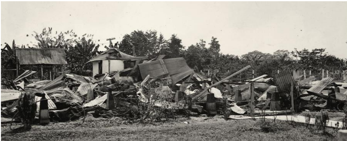
Figure 9. Engineers’ dormitories and machine rooms destroyed by demonstrators in Sevilla (Magdalena). Source: United Fruit Company photographic collection, box 30, No. 620. Photography taken on December 10 th , 1928. Publication authorized by Baker Library Historical Collections, Harvard Business School.
