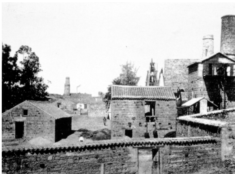
Figure 4. Linares Lead Mining Company Ltd., Pozo Ancho mine. The photograph was taken towards the end of the 19 th Century. The house of the 30 inches winding engine is on the right of the photograph. The engine house to the rear of it housed a pumping engine. There is a house for a set of roller crushers in the centre of the photograph, possibly also worked by the winding engine. (Colectivo Proyecto Arrayanes).
