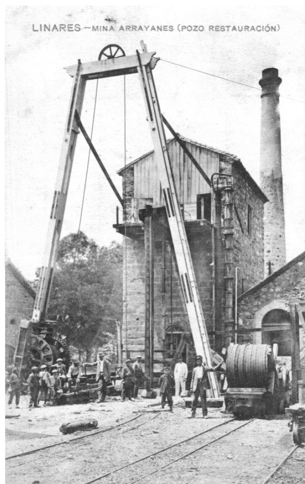
Figure 13. Restauración pumping shaft at the Arrayanes mine. A drum on the right of the photograph contains flat rope for use in winding (Author's Collection).
