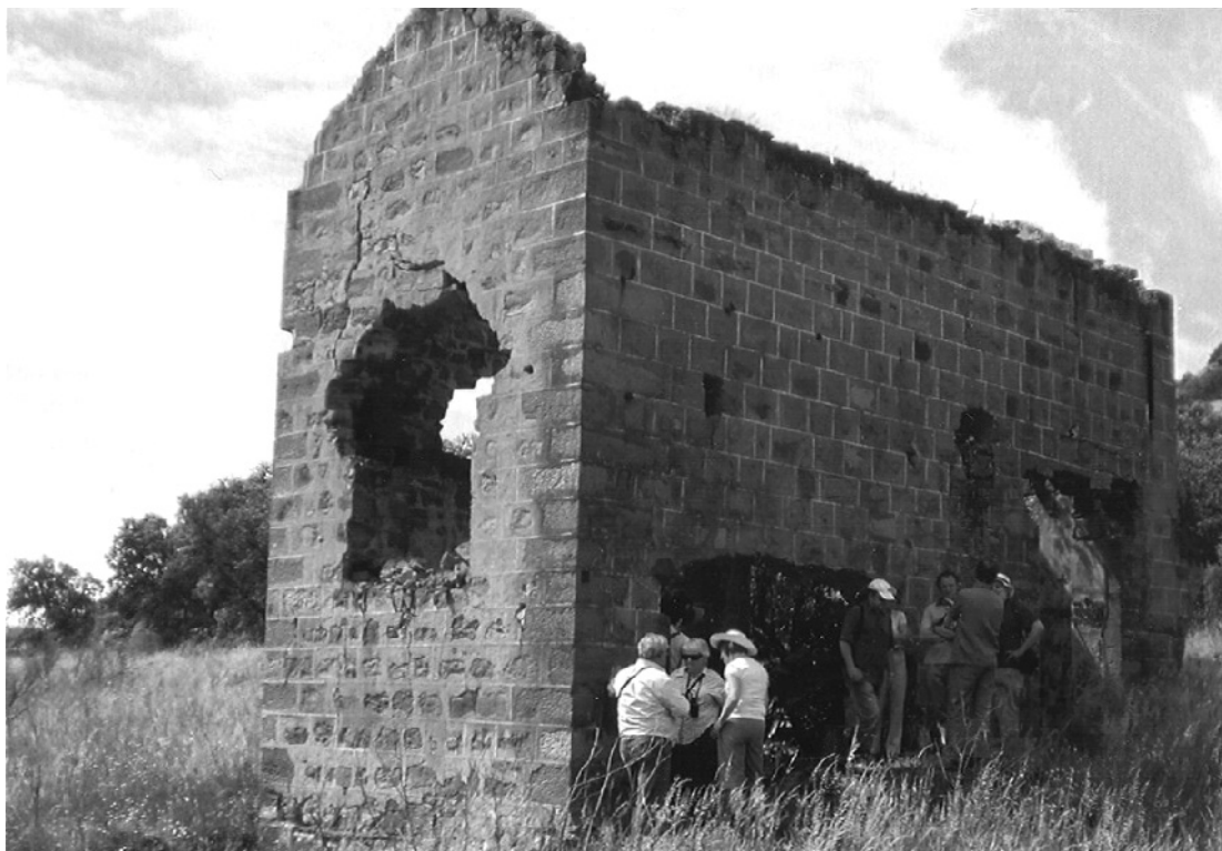
Figure 3. Pozo Briones: Early winding engine house. It enclosed a small beam engine. The opening in the wall between the groups of people was for the drive shaft to the winding drum that was located on the outside of the wall (Bob Barnes).
