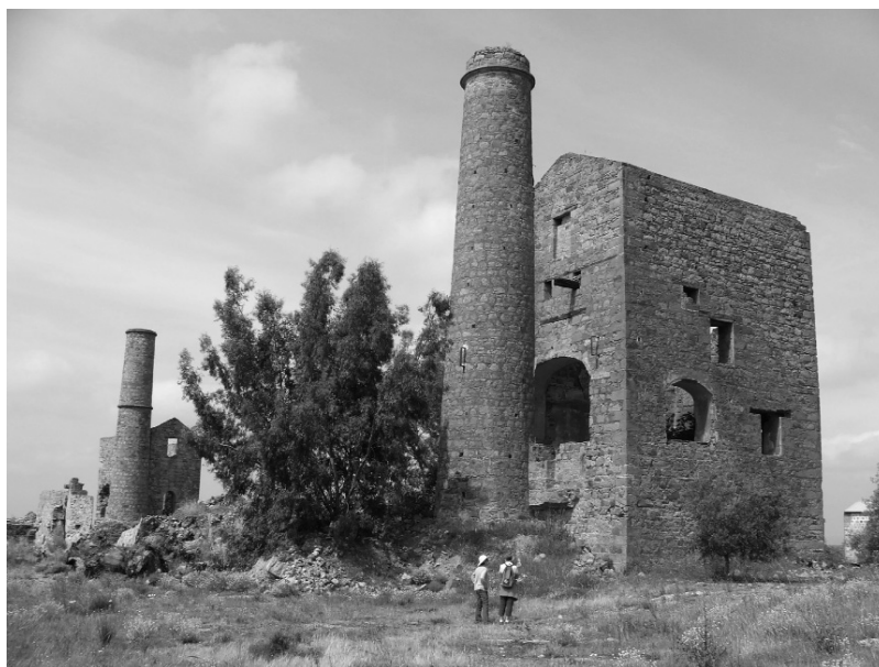
Figure 5. Linares Lead Mining Company Ltd., Pozo Ancho Mines, May 2009. The pumping engine house, with the winding engine house in the background (Author).
