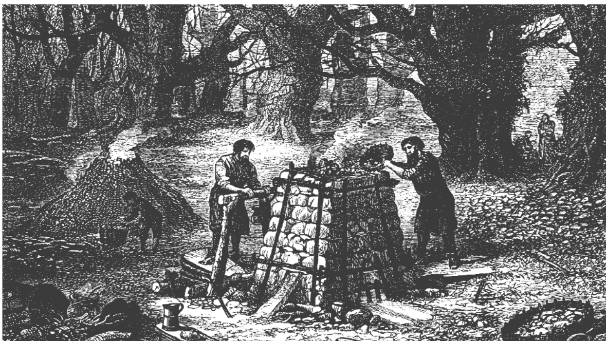
Figure 5. Primitive iron production in the forest. Note charcoal production in the kiln on the right and a worker operating a bellows.
